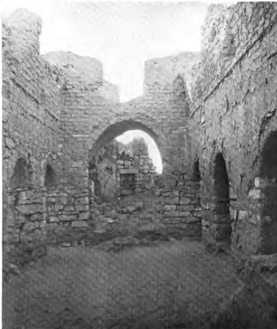
(c) Interior looking west.
